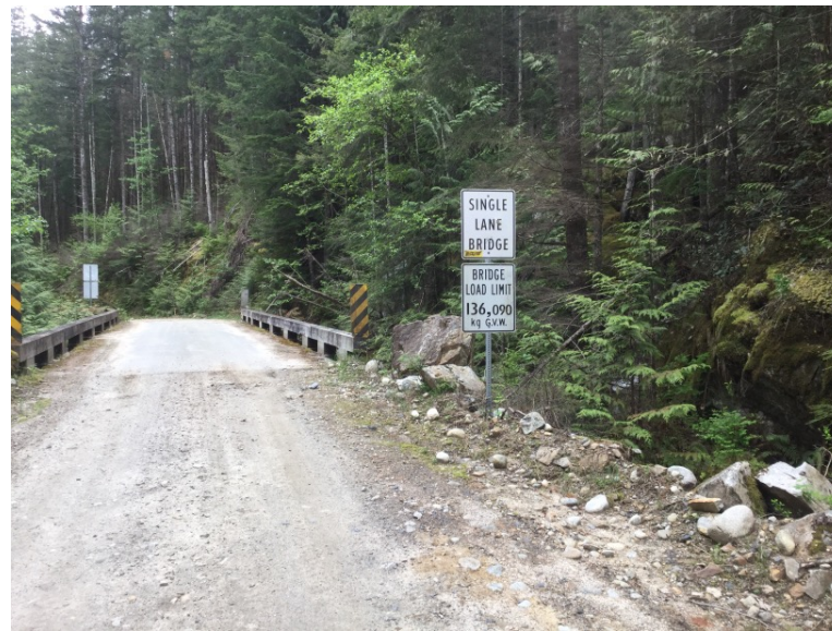
Load Rating Sign
