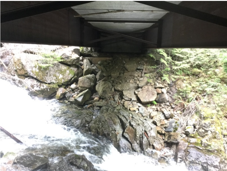
Left Bank Abutment when facing downstream
