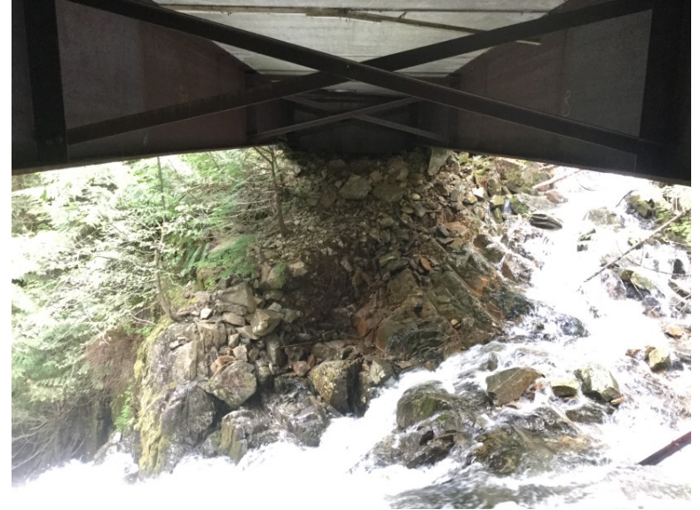
Right Bank Abutment when facing downstream
